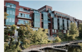
Ironworks Site After Utilizing TIF
