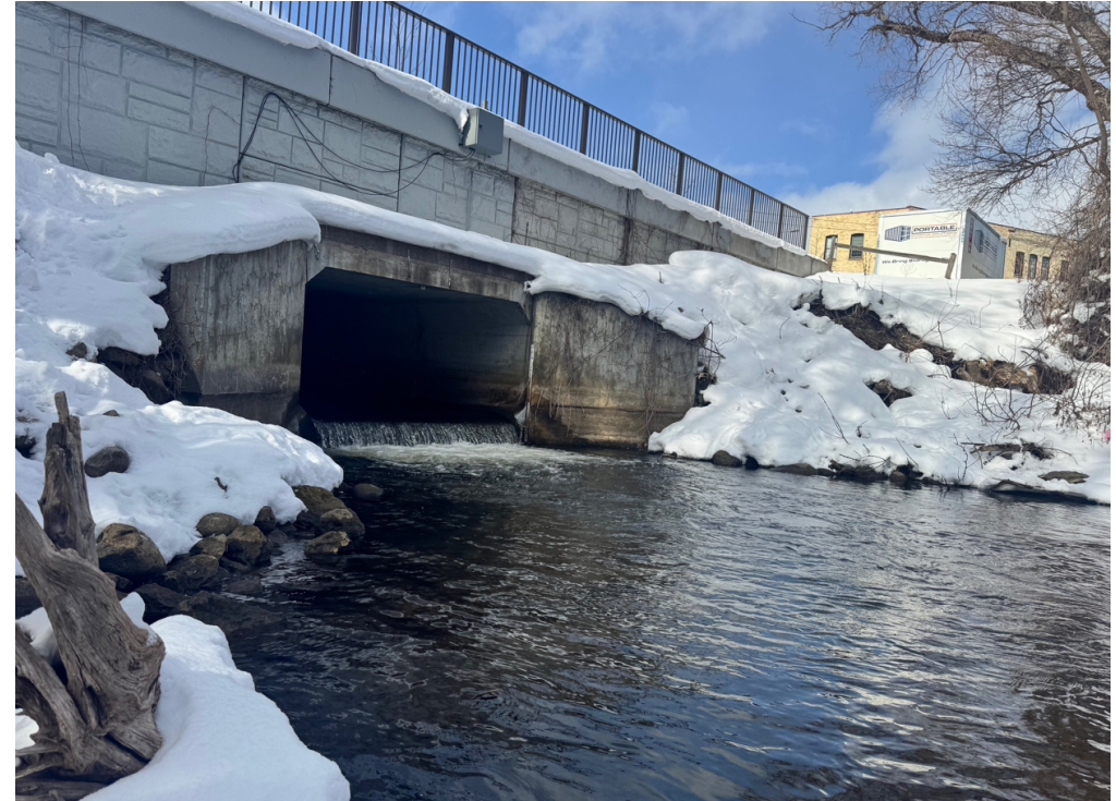
Existing Kids Creek Culvert
