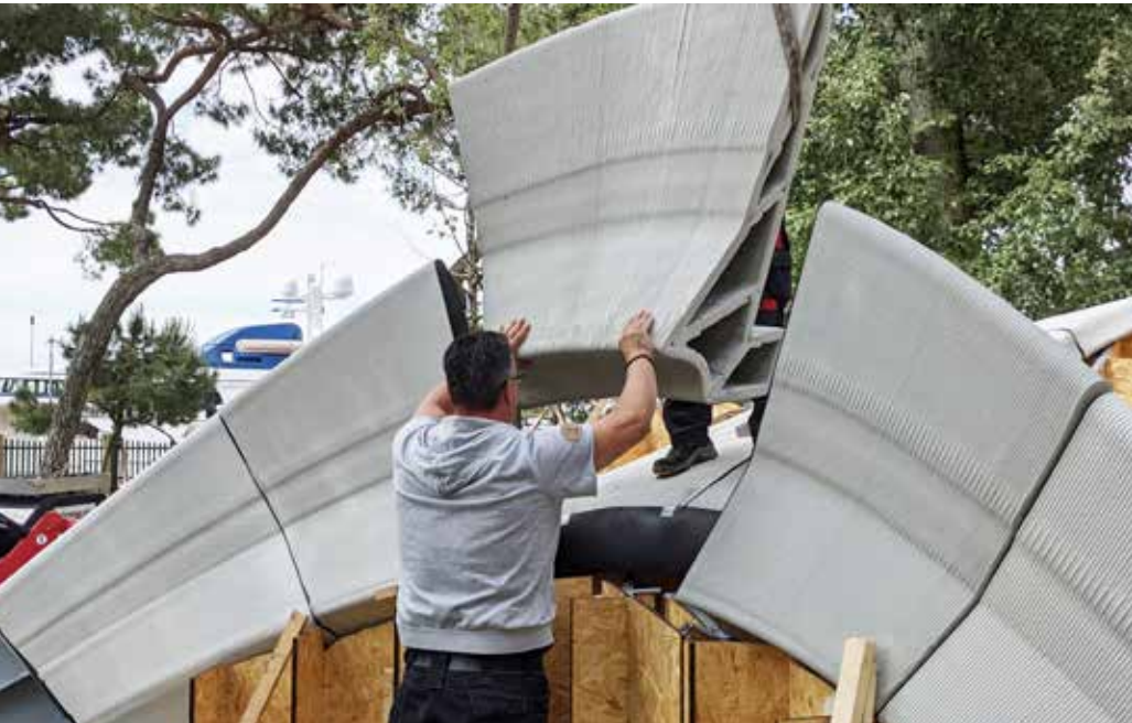
PRE-FABRICATED PEDESTRIAN BRIDGE COMPONENTS
